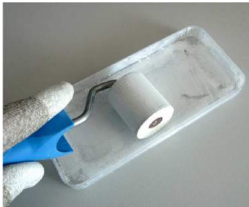
Figure 6: Working the paste onto the roller using a hard plastic tray
