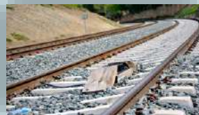
Track Obstacle Intrusion Inspection
